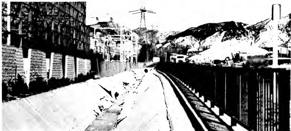
Photo 6. Left-lateral displacement in concrete culvert (view northwest) parallel to Sylmar Converter Station and Sepulveda Road. Produced either by underlying tectonic displacement on the Mission Hills fault or by an extensive landslide.
